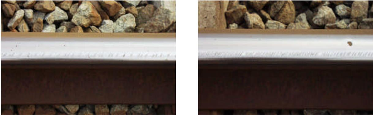
Figure 1: Headchecks at gauge corner
