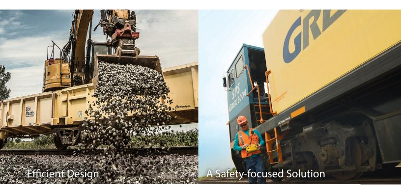
SlotMachine provides a continuous platform from which the excavator can work, so there's no pausing to switch out cars or reposition the crawler.
