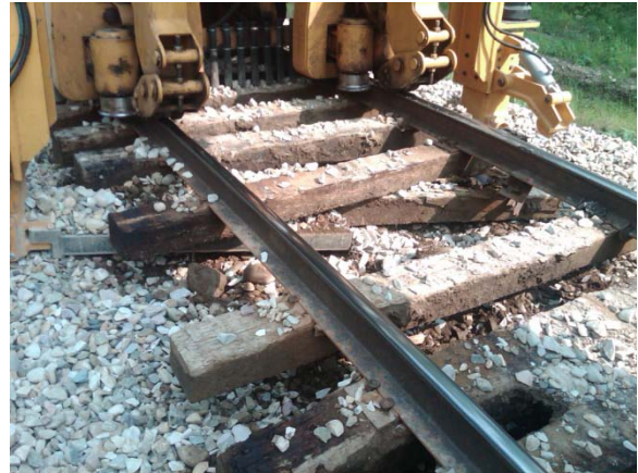
(Fig 9 - Dropped Tie on ANY Subdivision, 2010)
