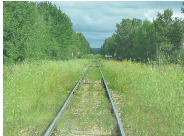
(Fig 2 - CN - ANY Inspection, 2008)
