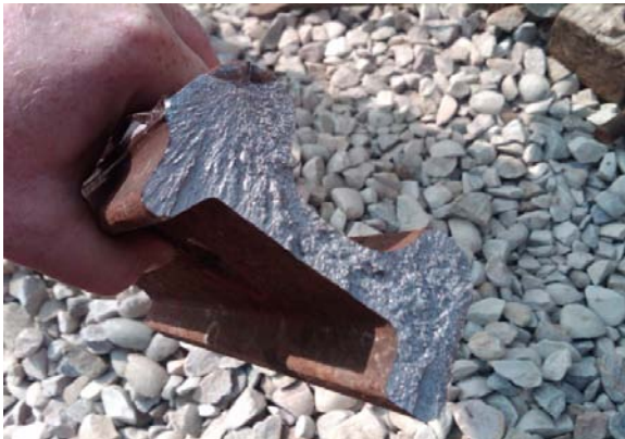
(Fig 13 - Defective joint bar on ANY, 2010)
