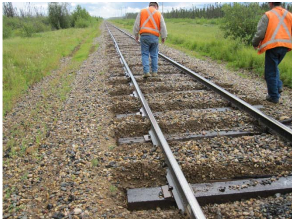
(Fig 6 -Ties replaced on the ANY, 2009)
