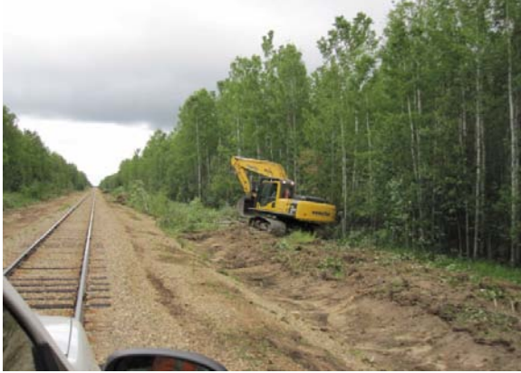
(Fig 8 - Drainage work on the ANY, 2009)
