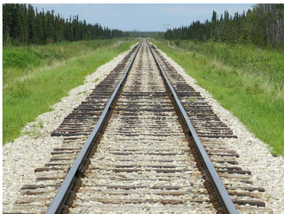
(Fig 7 - Ten foot ties in muskeg soil area)
