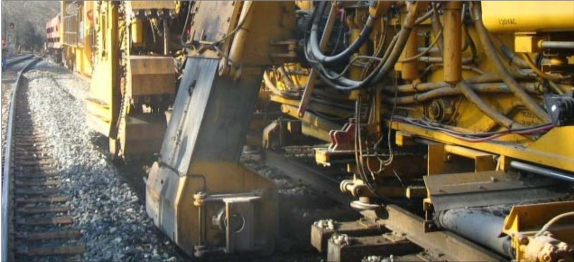
**Figure 7. Track Undercutting<sup>3</sup>**
