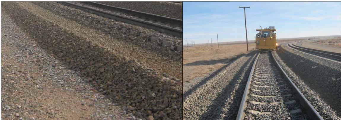
**Figure 5. Shoulder Cutting to Improve Drainage**
