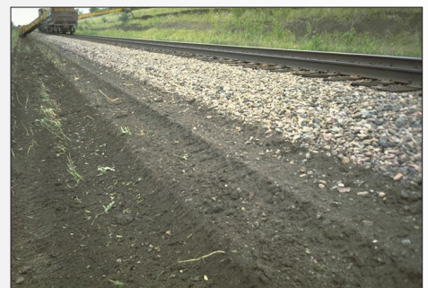
Finished ditch directs water away from track structure where it can drain and evaporate.
