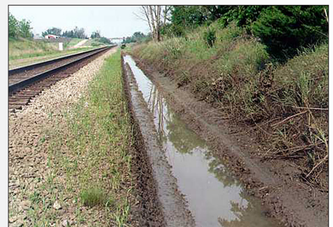
Trapped water revealed after ditch is cut.
