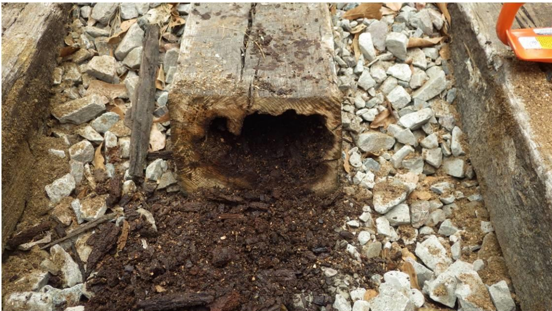
Figure 9: Tie surface and subsurface after destructive examination. The void is readily apparent.
